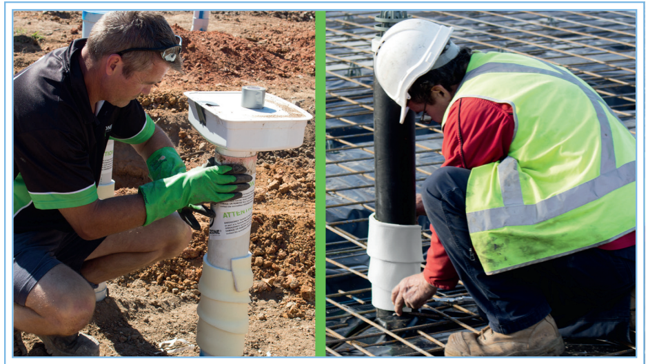
Greenzone can be installed before formwork (left) or after formwork (right)
